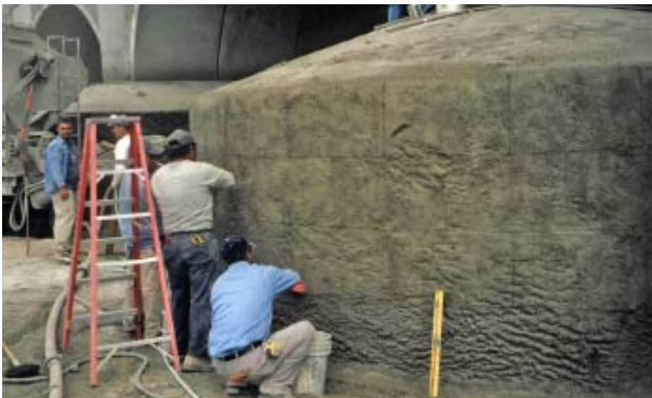
After the application of a shotcrete layer on the face of a concrete pier of the bridge, workers cut grooves in the partially set material to give the surface the appearance of cut stone.
