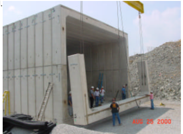
Bottom 3-sided unit being set into position.
