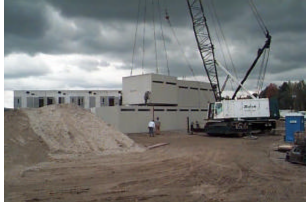
Cell module being erected in one of the 5 housing pods.
