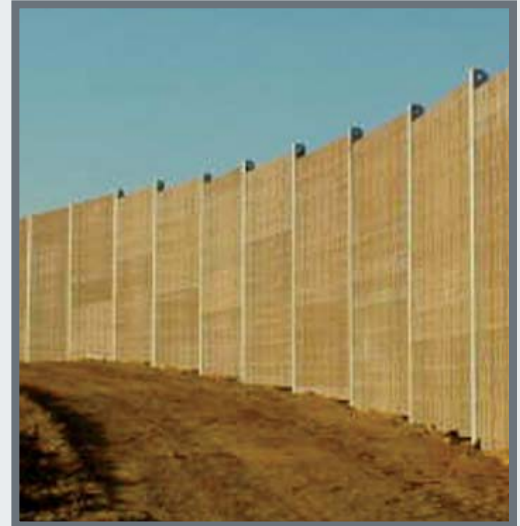
Precast Noise Wall
